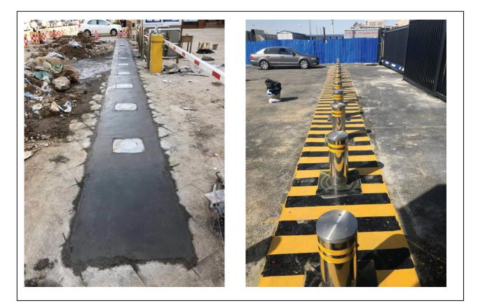
Step 7: If the bollards work well, fill the concrete to fully fix bollards. After the concrete dry, you can also paint the surface of the road so it will be easier to be notice.
