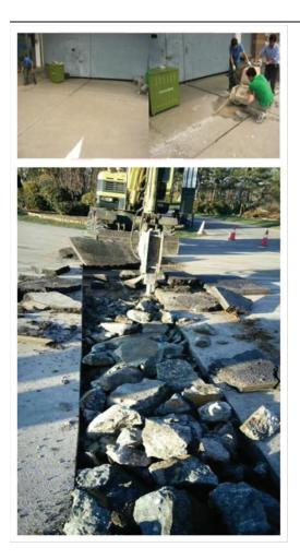
Step 1: According to the construction drawings given by the manufacturer, dig the groove trough, lay the foundation, and do the drainage; ensuring that the 220V power supply is connected to the construction site; pre-bury the required pipes and wires.
