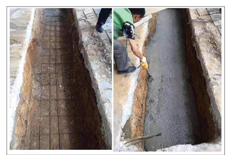
step 2: Layout the concrete base at the location of where you place the bollards
