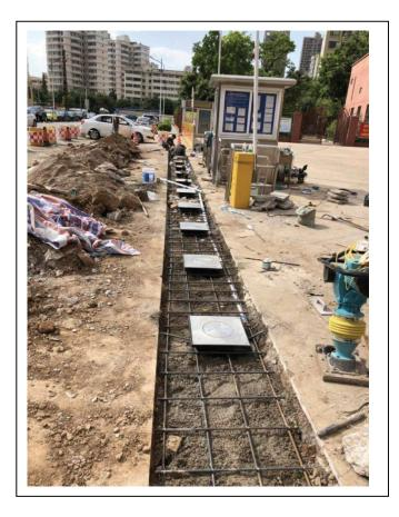
Step 4: Fix in the concrete or asphalt to fix the bollards. Note:Please cover the bollards with some protective film. Do not let concrete and sand or other objects penetrate into the bollards body! If some big object penetrate into the casing of the bollards,it will affect the operating of the bollards. It may get stuck or cannot be up and down fully.please pay attention to that.
